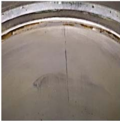
Examples of bore discoloration
