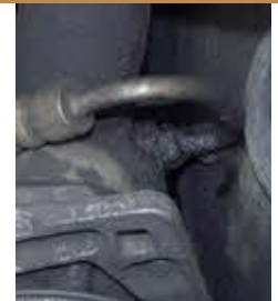
Power steering leak at pump
