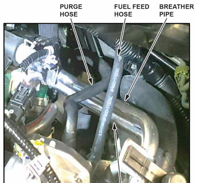
No good condition: Fuel feed hose and purge hose routed over the breather pipe.
